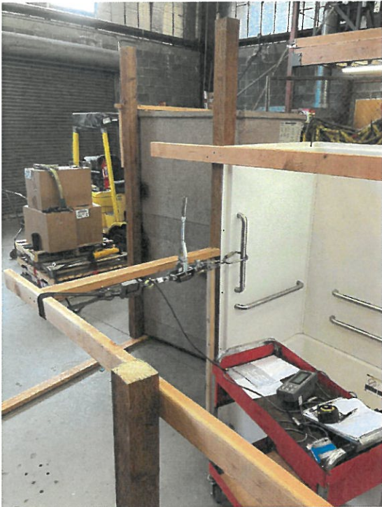
Photo 5 - Horizontal Test at Location C
