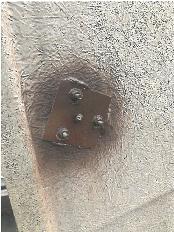
Photo 16 – Factory installed nuts and washer
