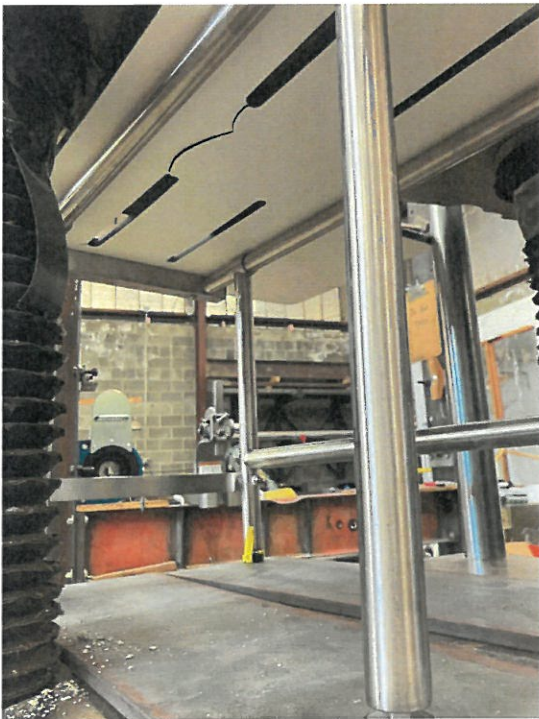
Photo 15 – Crack developed at failure of seat with 5" by 15" bearing plate
