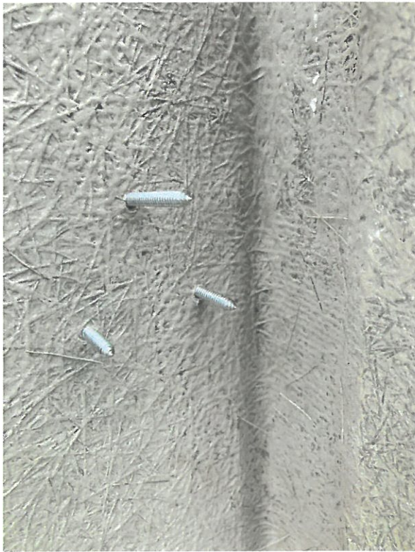
Photo 17 – Field installed wood screws
